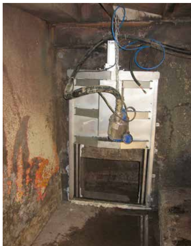
Sluice gate valve under paint booths
